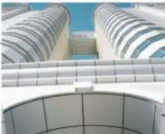
■ Soffits and Beams
